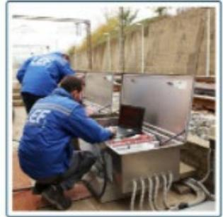
A G3-PLC installation used for tunnel safety offers to monitor emergency lighting switch on, the status of the push-buttons and the power consumption of each lamp, with alerting in case of anomaly detection.
